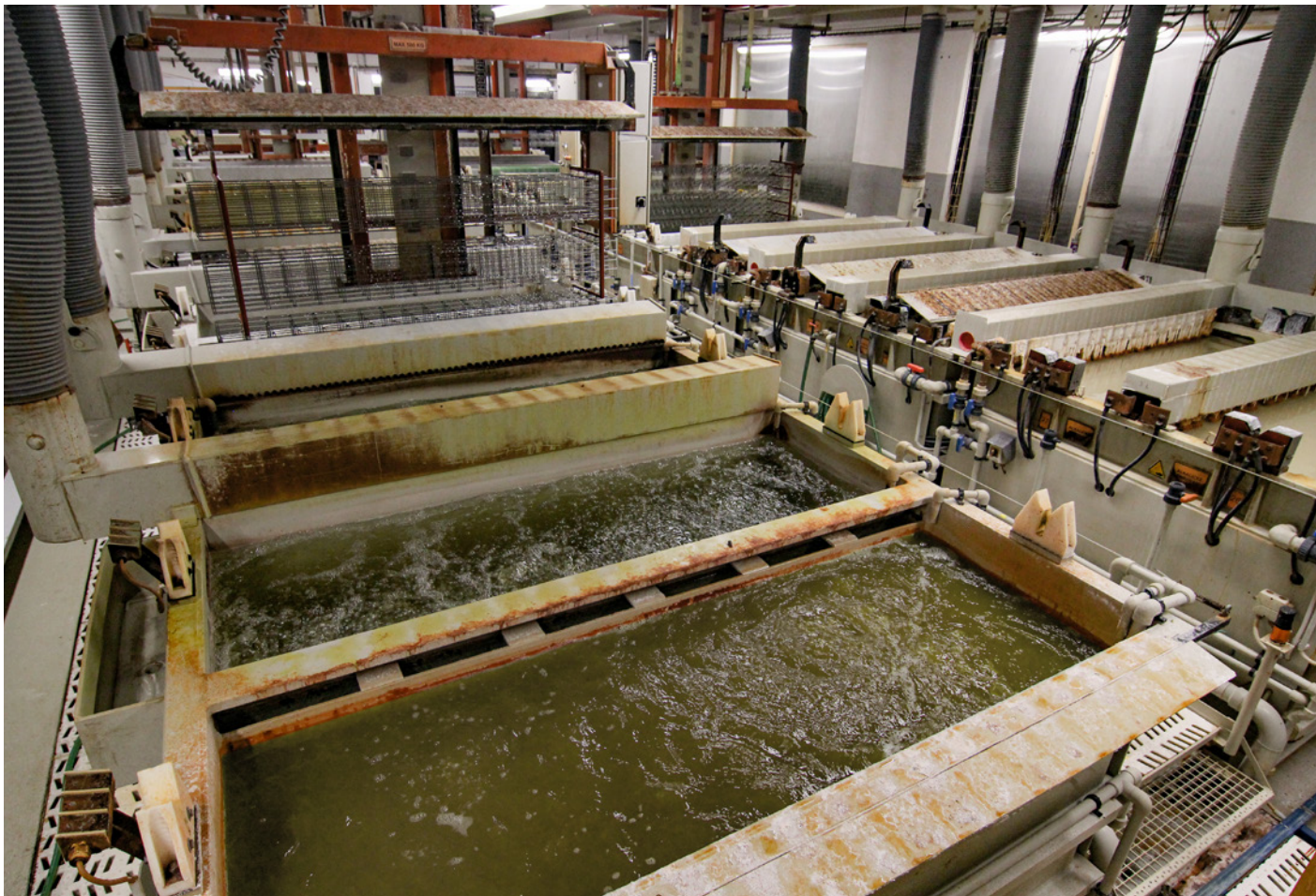
▲ Galvanizing line in the production premises in Uhřetice.
